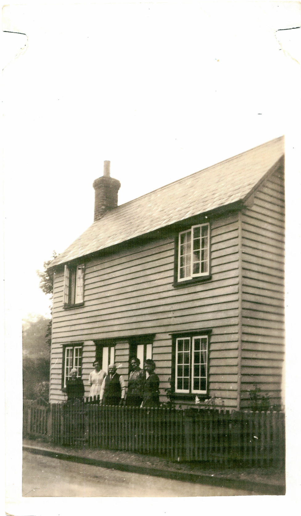
FIRS COTTAGE HEMPSTEAD.
